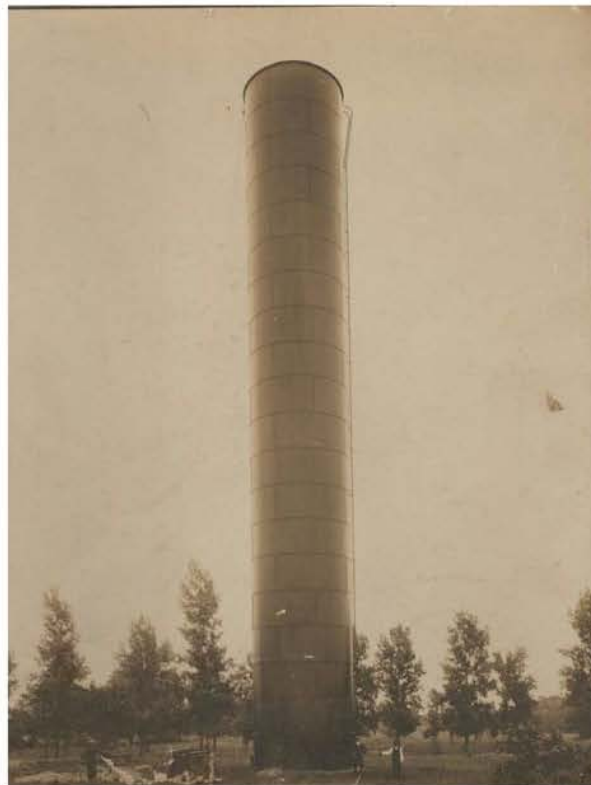
Wenonah's 100-foot high standpipe.
